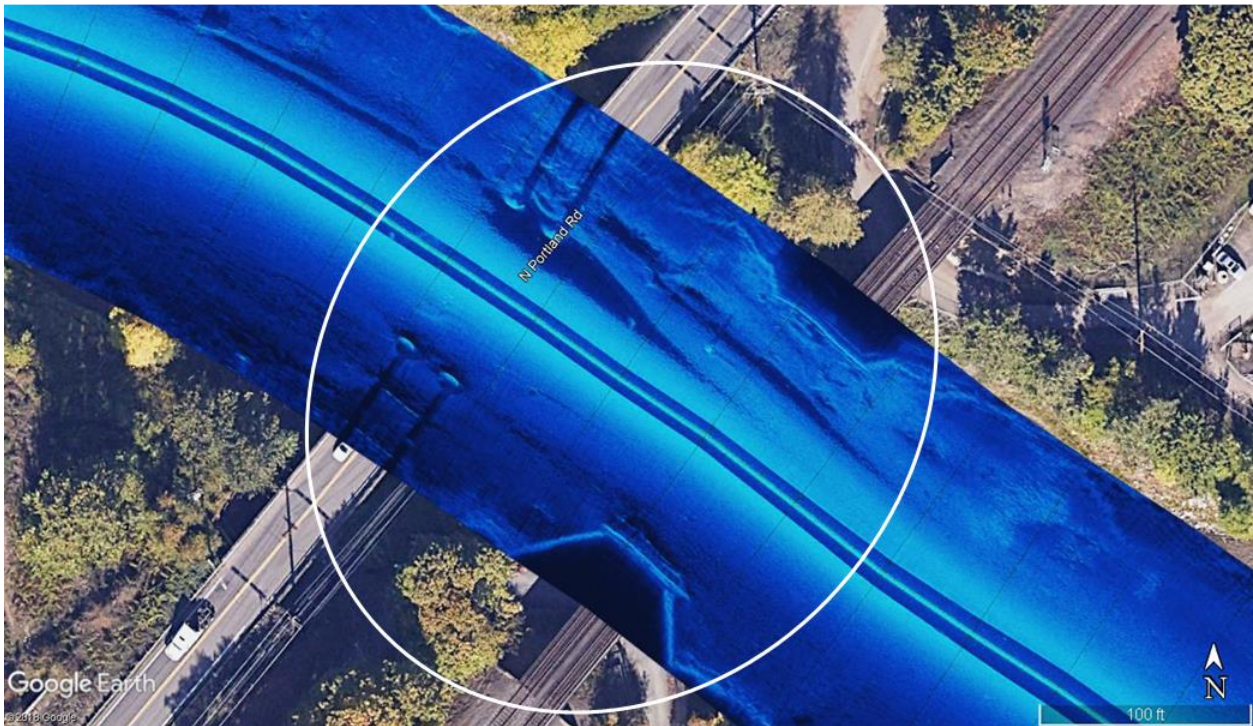
Reach 1 bridge structure; the various types of supporting foundations for bridges can be seen in Reach 1. These include North Lombard Street near North Kelley Point Park Road (top), and a bridge on North Portland Road and its neighboring railroad bridge (bottom).
